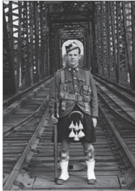
On guard at the railway bridge over the Burlington Bay Canal, 1940.
